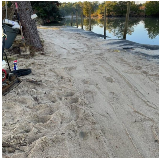
Figure 8: Recently permitted and constructed project utilizing geotubes filled with dredged material in Gloucester. The picture shows the tube as it is being covered with sediment. Grass has since been planted atop the tube and the site will function as a docking area at a public boat landing.
