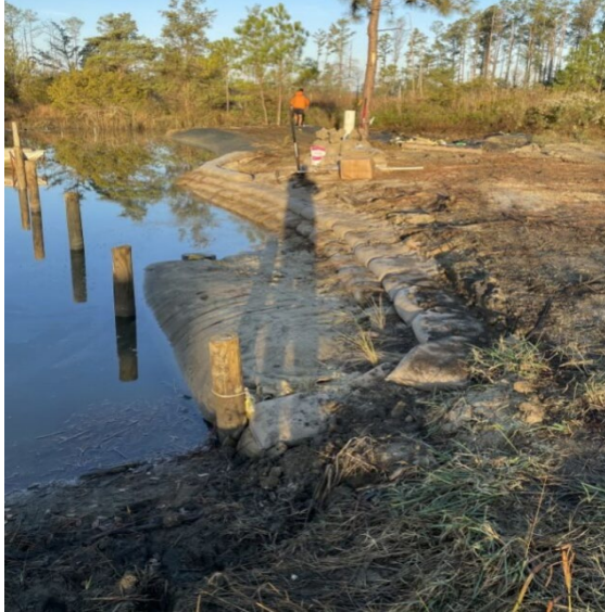
Figure 5 (above): Recently permitted and constructed project utilizing geotubes filled with dredged material in Gloucester. The tube has been covered with sediment and tidal marsh grasses have been planted atop the tube as part of a living shoreline.
