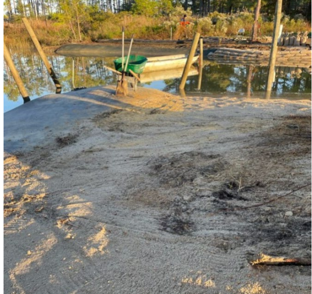
Figure 6 (above): Recently permitted and constructed project utilizing geotubes filled with dredged material in Gloucester. The picture shows the tube as it is being covered with sediment. Grass has since been planted atop the tube as part of a living shoreline.
