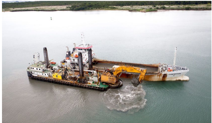
Figure 12: Example of In-Water Dewatering via mechanical dredging and placement within a hopper dredge (from IADC Dredging).
