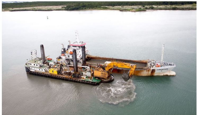
Figure 12: Example of In-Water Dewatering via mechanical dredging and placement within a hopper dredge (from IADC Dredging).
